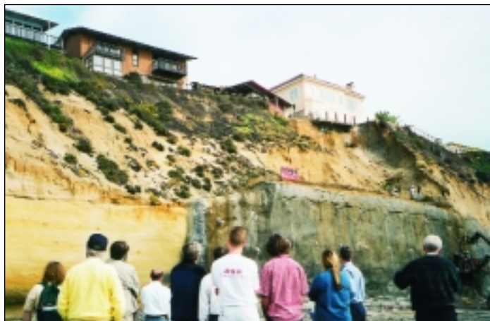
Conference participants had a chance to view eroding see cliffs with active landslides on the Bluffs and Seawalls field trip organized by Walter Crampton of Terracosta Consulting Group, Inc. Various types of seawalls and retaining structures are in place to prevent cliff erosion. The one pictured here is being constructed by JC Baldwin Construction Company, one of the conference exhibitors.
